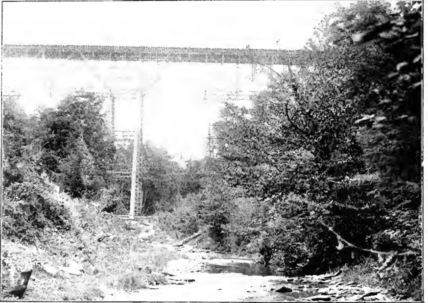
MILL CREEK BRIDGE—115 FT., Dansville, N. Y.
